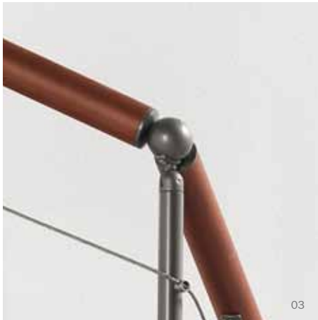
03 _ Handrail metal connection joint.
